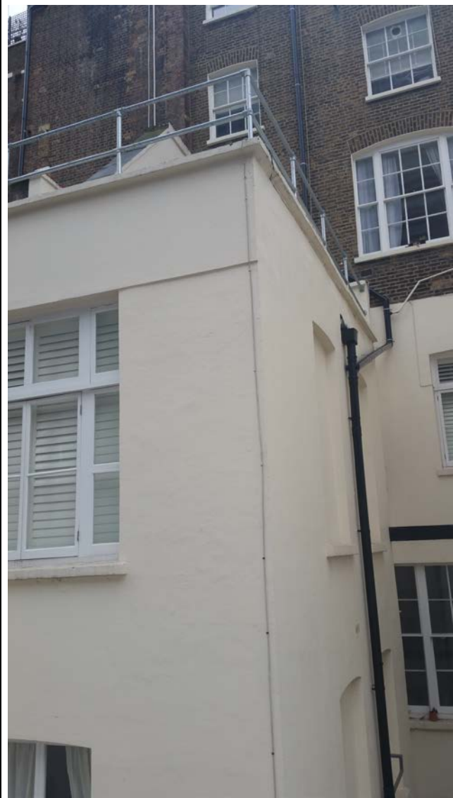
VIEW FROM FIRST FLOOR LEVEL OF 101 EASTBOURNE MEWS LOOKING OUT TO 101 WESTBOURNE TERRACE.
