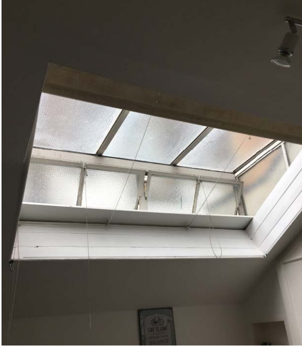
Existing first floor glazing to rear bedroom
