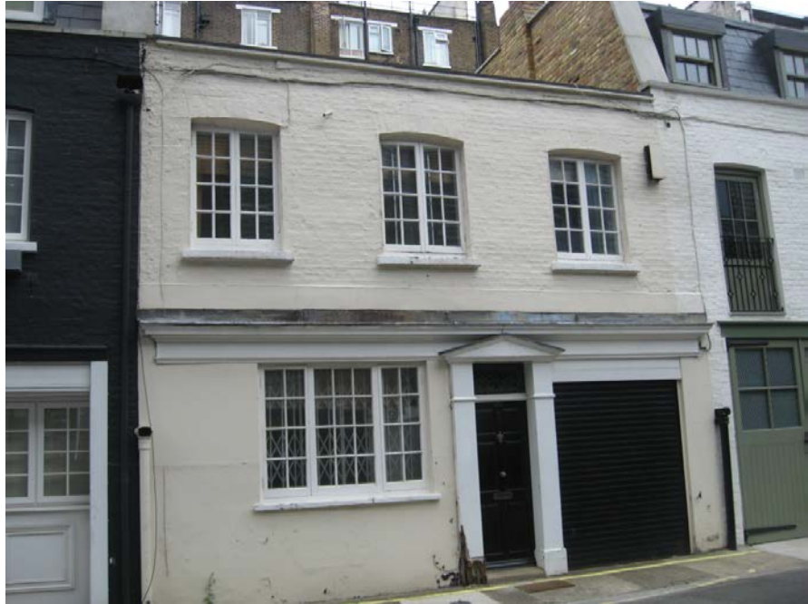
Application site, 103 Eastbourne Mews, front elevation
